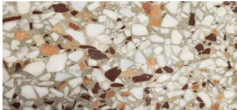
EXISTING TERRAZZO FLOOR
