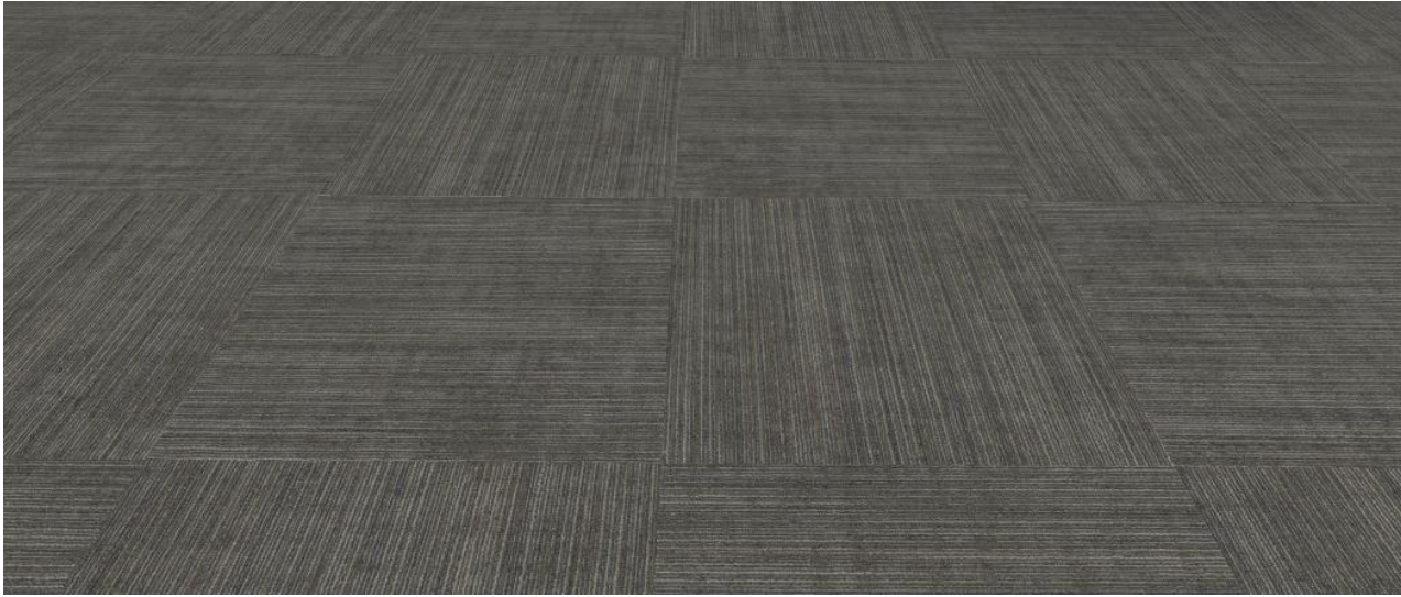
CARPET TILE INSTALLED
